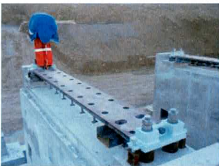
Figure 13. Main housing frame
