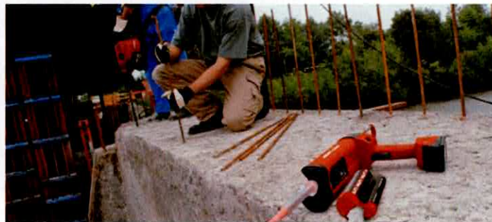
Figure 21. Chemical anchor
