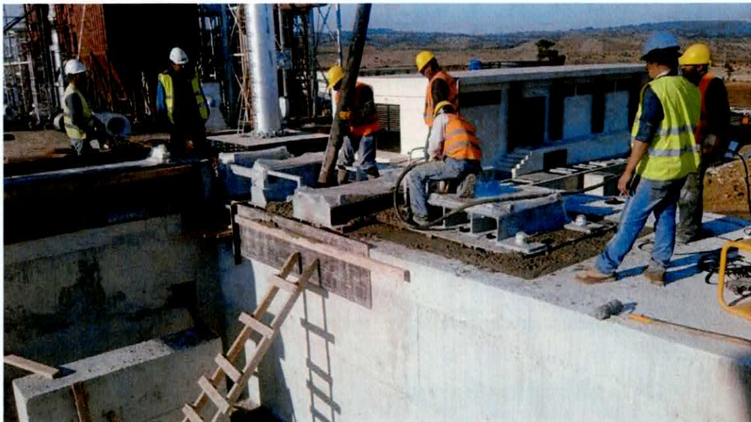
Figure 20. Concrete puring
